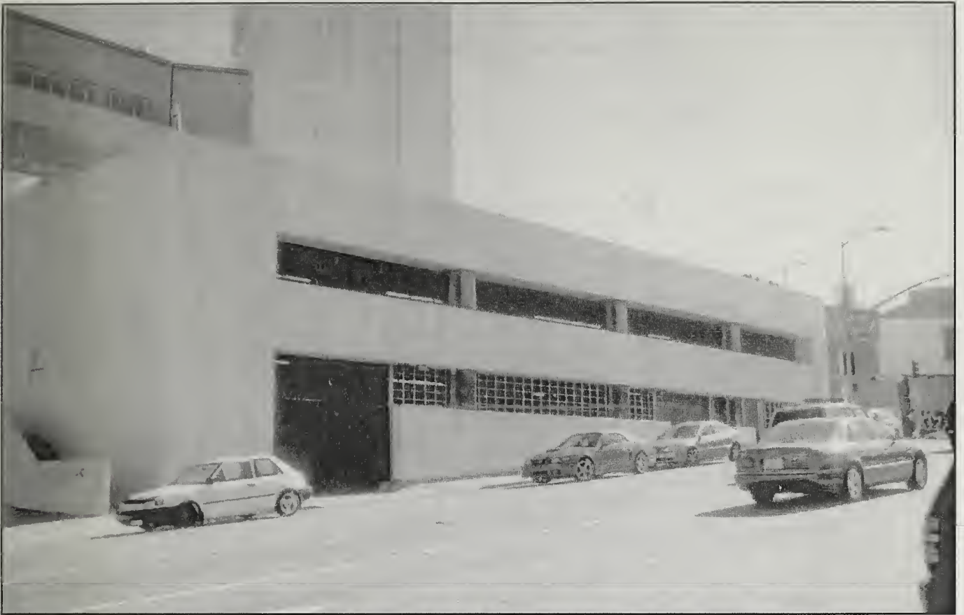
Figure 44 - Parking Structure North Facade (Harrison Street)
